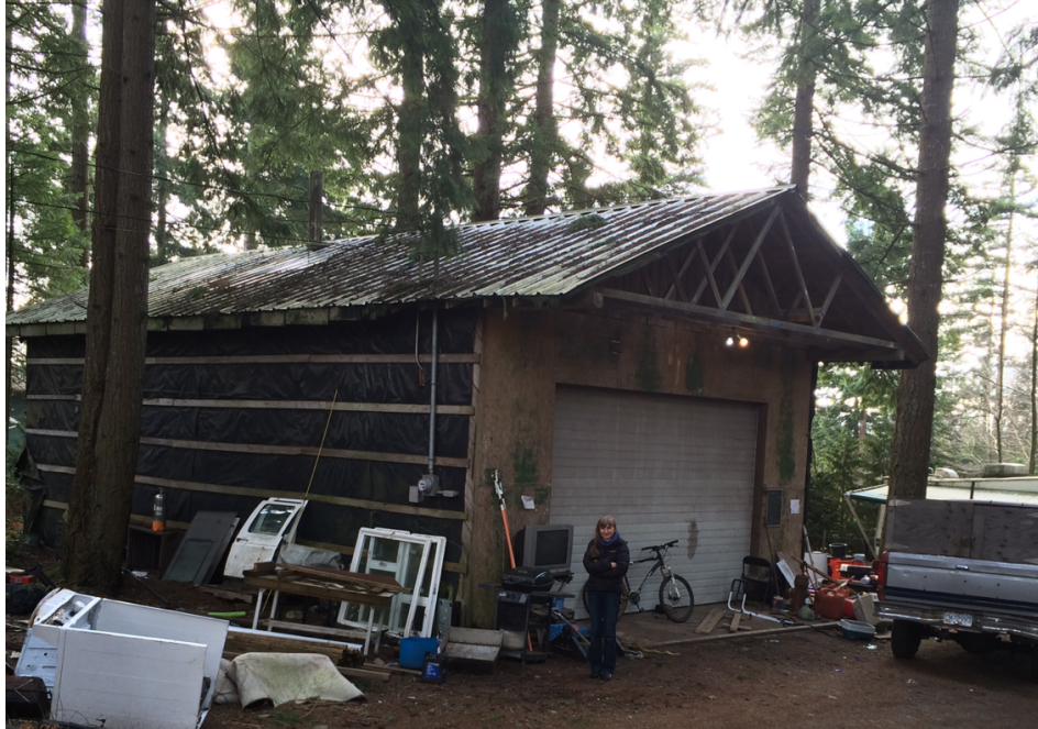
7413 North Island Hwy workshop pre- renovation N. W. corner May 2015
