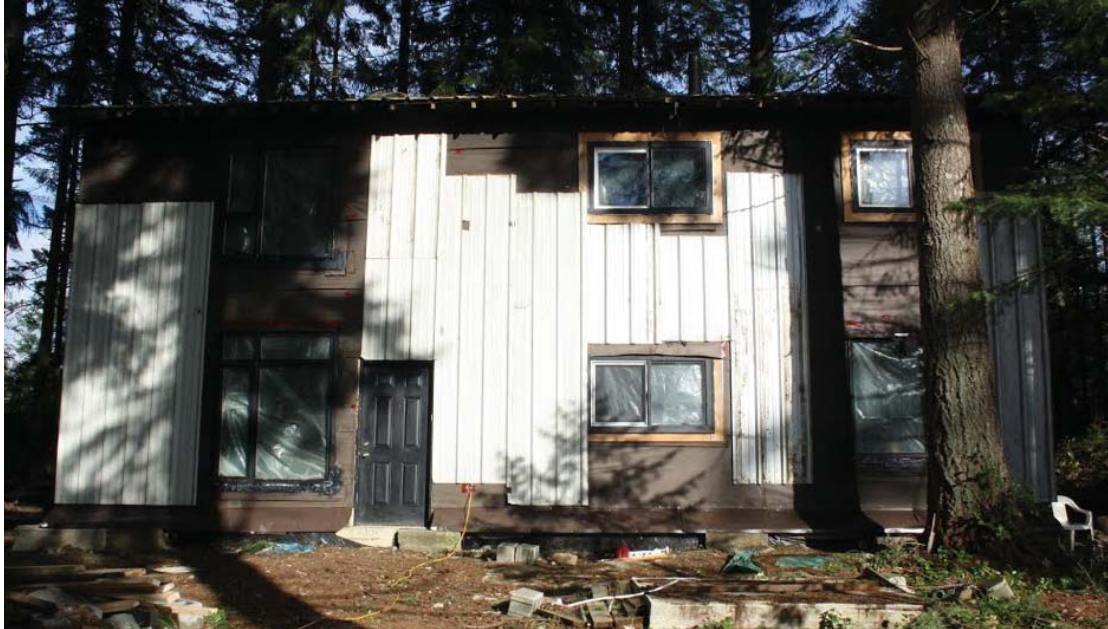
South side view Nov 2016 a portion of original siding replaced as rain shield
