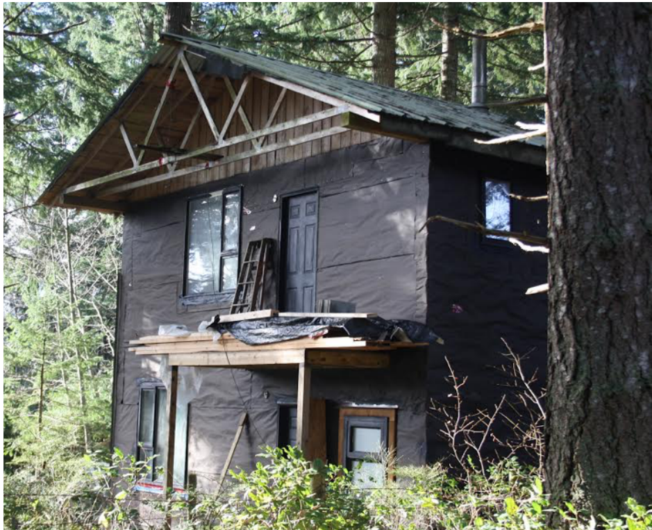
7413 North Island Hwy workshop with renovation N. E. corner Nov. 2016
