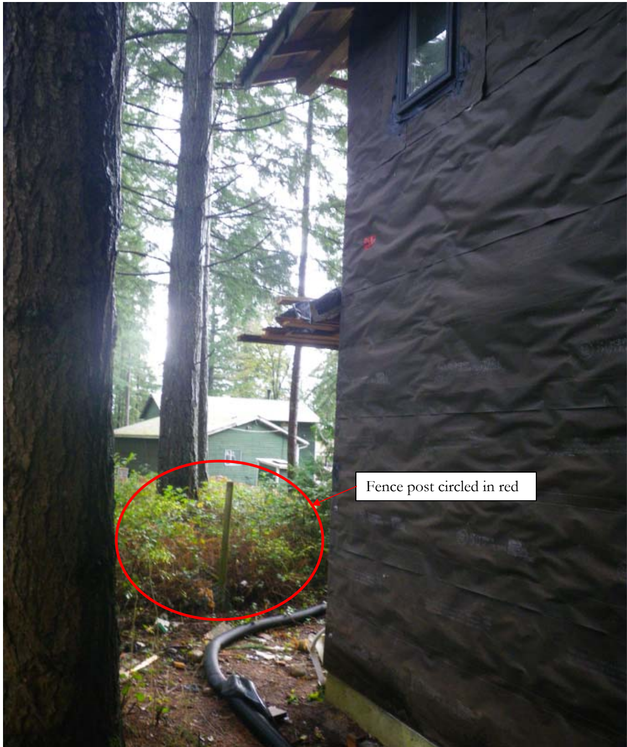
Figure 4: View of Neighbouring Property, Distance Between end of Accessory Building to Fence Line
